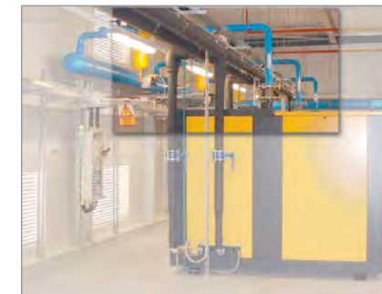
Fig. 3b: Vibration-dampening compressor connection with axial compensators
