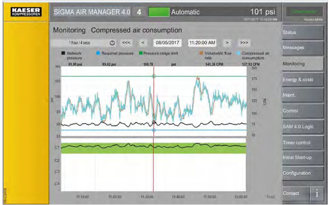
Fig. 111 Menu Monitoring – Compressed air consumption
