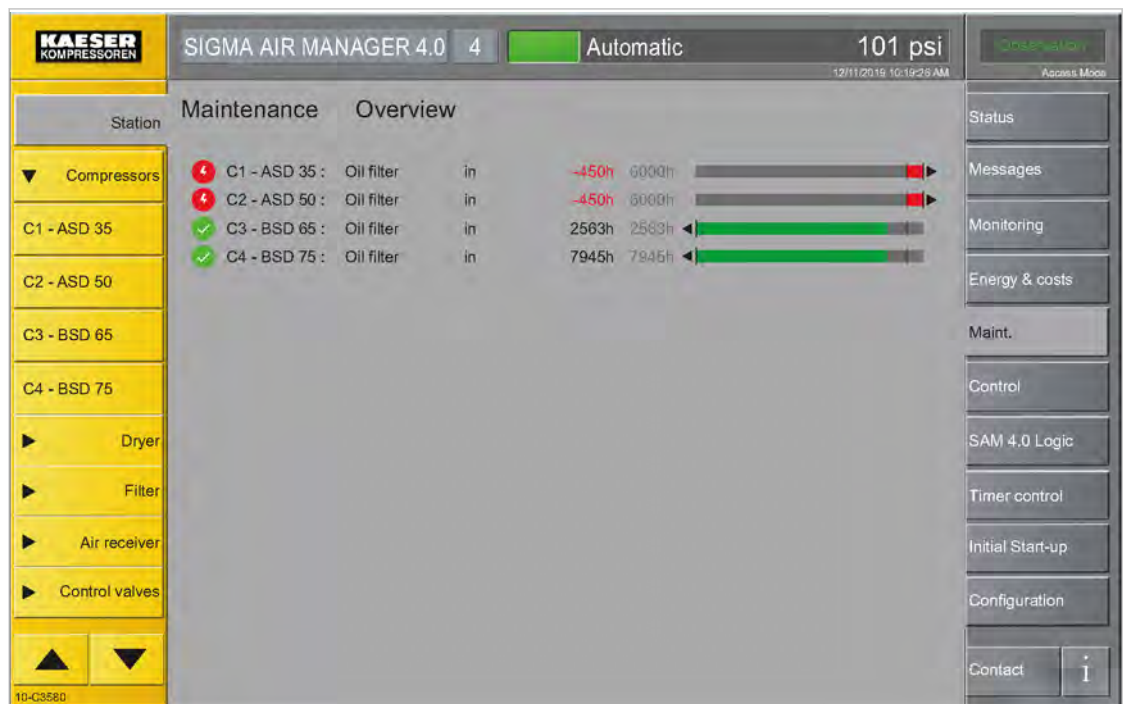
Fig. 132 Menu Maintenance – Overview for the entire station
